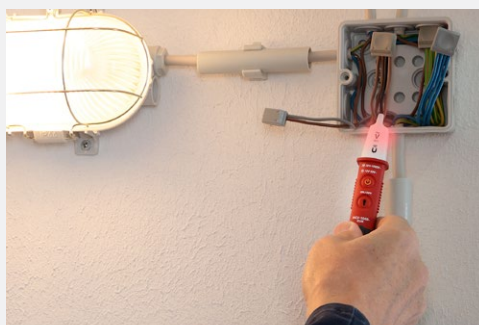
Test wires for AC voltage for quick troubleshooting
