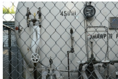
Difficult inspection sites
